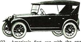
1922 - America's first car with the engine mounted on rubber to defeat vibration.
