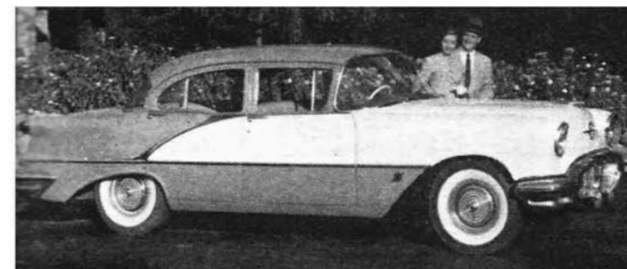
Super 88 4-door sedan has its own distinctive side trim and sports same 240-horsepower Rocket engine as 98. Note stylish tear-shaped fender cutouts
