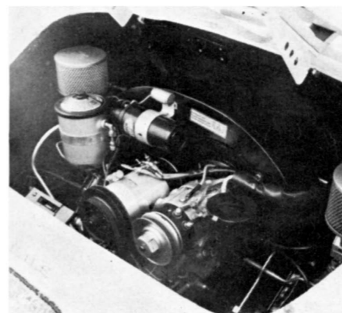
Extra generator mounted at left of regular generator supplies auxiliary batteries with power for short wave set.
