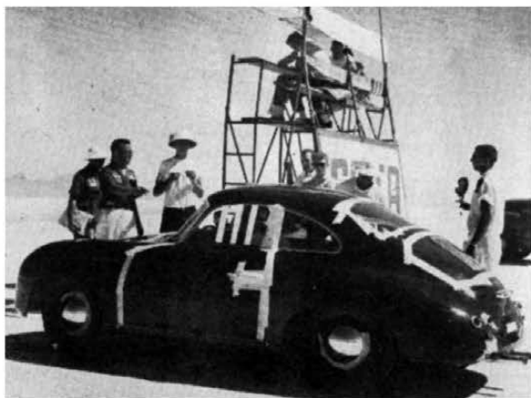
This Porsche Carrera coupe, entered by Ralph Duke Stewart, turned a best time of 115.53. Again masking tape helped to cut turbulence in window and door spaces.
