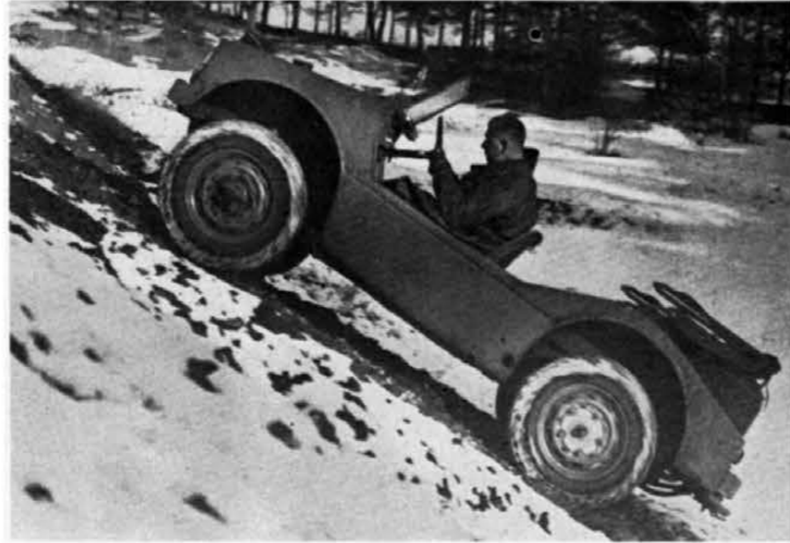
All four wheels spinning, the Jagdwagen charges up a mud and snow covered slope. Slants of 65% are possible.
