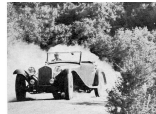
In fast turn, front wheels follow any curve on rails; rear wheels slide out until they align with front, then sliding always stops.
