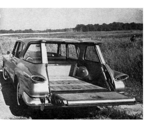
**FOLD-DOWN** tailgate features roll-down rear window with power operation standard on three-seat and optional on two-seat models. Rubber bumper steps ease entrance to rear.
