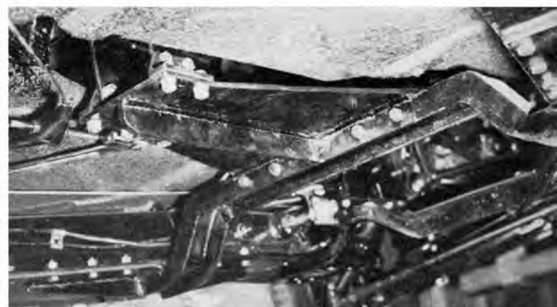
Viewing same area shown in photo above, this time from below, reveals welded-up, bolted-in special rear crossmember supporting rear end of transmission and engine assembly. Trans is Corvette 4-speed unit, rests on crossmember through stock mount. 3/32-inch wall steel tube driveshaft has Chev and Stude U-joints.
