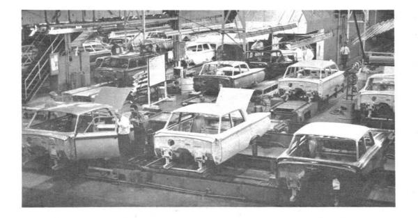
Fully painted bodies are placed on a floor conveyor and moved into the storage and inspection area. After a thorough, last-minute inspection they will enter the tributary known as the trim line. At the station shown here, the body, insofar as the welded joints, interior and exterior paint and general appearance are concerned, is finished. Any corrections needed on door and deck lid fittings will be made on the final assembly line.
