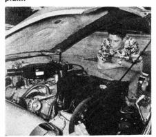
Although four-speed manual transmission takes up more space than previous boxes, installation is neat.
