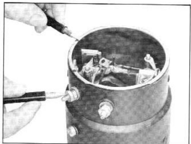
Fig. 13-33 Checking Positive Terminal for Ground
