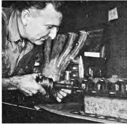
Match ports to manifold and smooth them out. Don't enlarge them; you can't increase manifold same amount.
