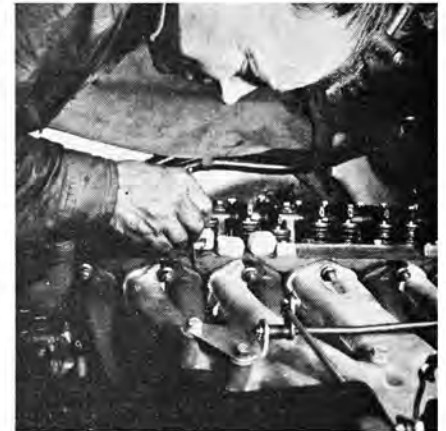
Cut wooden blocks to fit ports and use them to align manifold and ports. Then centerpunch manifold and head outsides for reassembly alignment.
