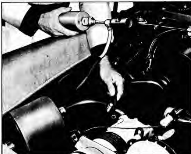
Fig. 5-40 Checking for Refrigerant Leaks
