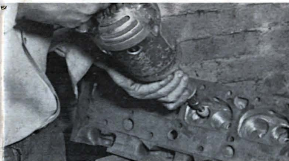
ABOVE—A cutter of this type can be used to enlarge the upper ends of valve ports for oversized valves.
