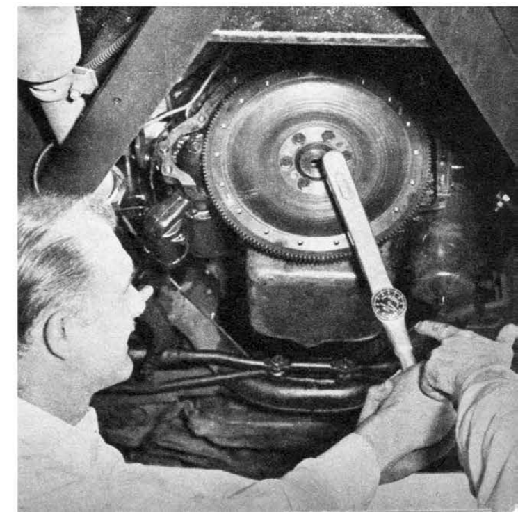
Installation of Hydramatic in Chevy requires grease rack or lift and hydraulic jack, is comparable to refitting of gearbox.
