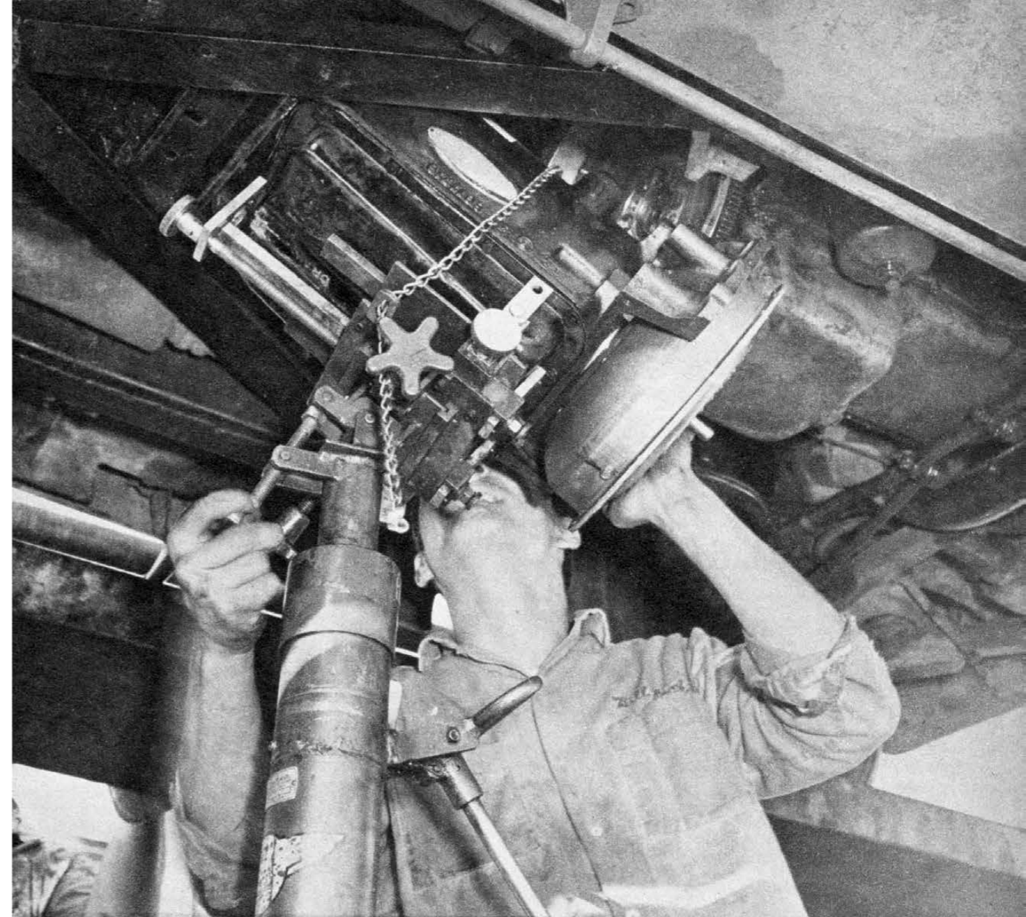
Installation of Hydramatic in Chevy requires grease rack or lift and hydraulic jack, is comparable to refitting of gearbox.
