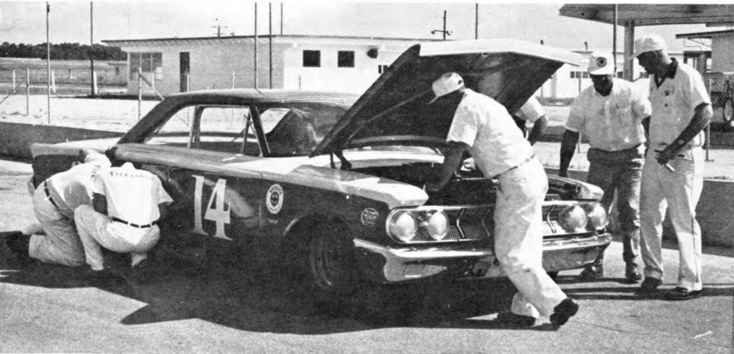
Special pre-season tests with prototype racing Mercury proved that new fastback roof line and "427" Marauder engine had potential to average 160 mph around Daytona Speedway.
