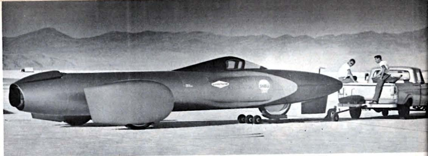
Craig Breedlove's Spirit of America is a huge machine aimed exclusively at land speed records. It has been troubled so far by the lack of good steering controls. Small fin at the bottom of the nose was meant to guide the car at high speeds. Its failure has led to need for steerable nose wheel.
