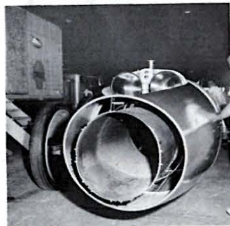
Craig Breedlove's Spirit of America is a huge machine aimed exclusively at land speed records. It has been troubled so far by the lack of good steering controls. Small fin at the bottom of the nose was meant to guide the car at high speeds. Its failure has led to need for steerable nose wheel.
