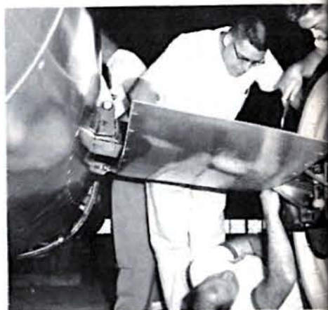
Craig Breedlove's Spirit of America is a huge machine aimed exclusively at land speed records. It has been troubled so far by the lack of good steering controls. Small fin at the bottom of the nose was meant to guide the car at high speeds. Its failure has led to need for steerable nose wheel.
