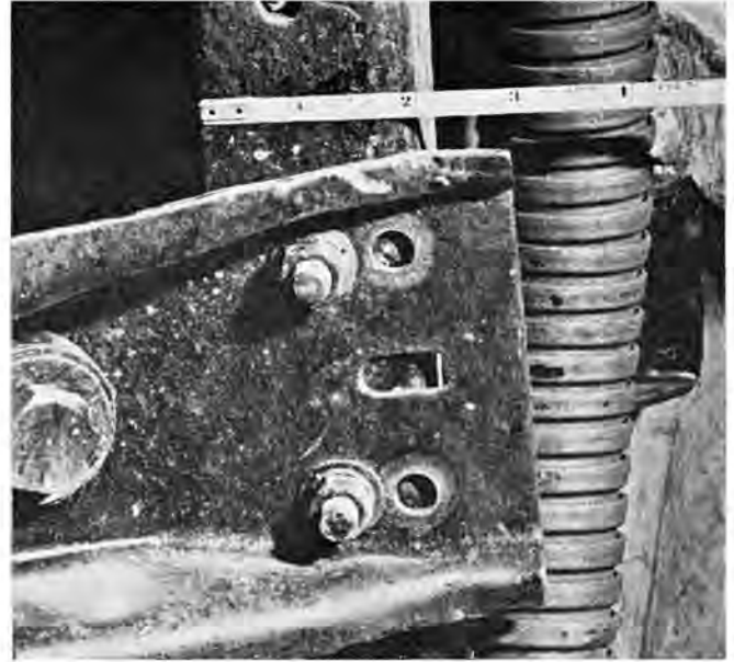
The distance between the bolts that secure the rear motor-mount crossmember's right end to the frame and their original holes shows how much the member was moved (about 3/4 inch) to provide clearance for the new engine.
