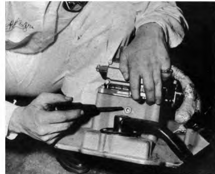
Out comes the smog-control paraphernalia. The manifold is plugged up, too.
