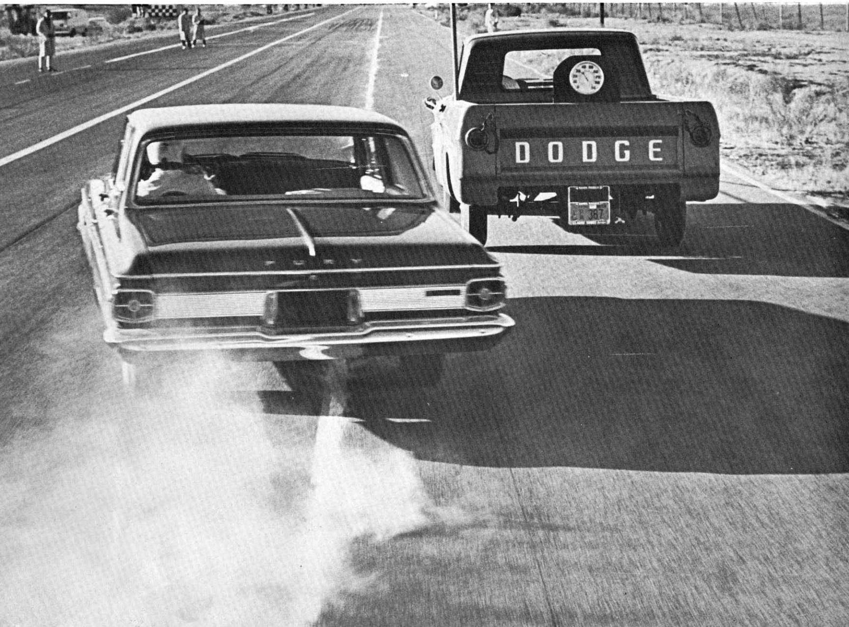
the chalk line for each car. The same procedure is followed for the Highway Passing Test, except that this time the test cars must pass the pace truck traveling at 55 miles per hour. In both passing tests, the cars were run individually with the drivers once again rotating to eliminate the human element. As you can see from the official average results, Plymouth won both passing tests, demonstrating a remarkable combination of immediate response and positive handling so necessary for
