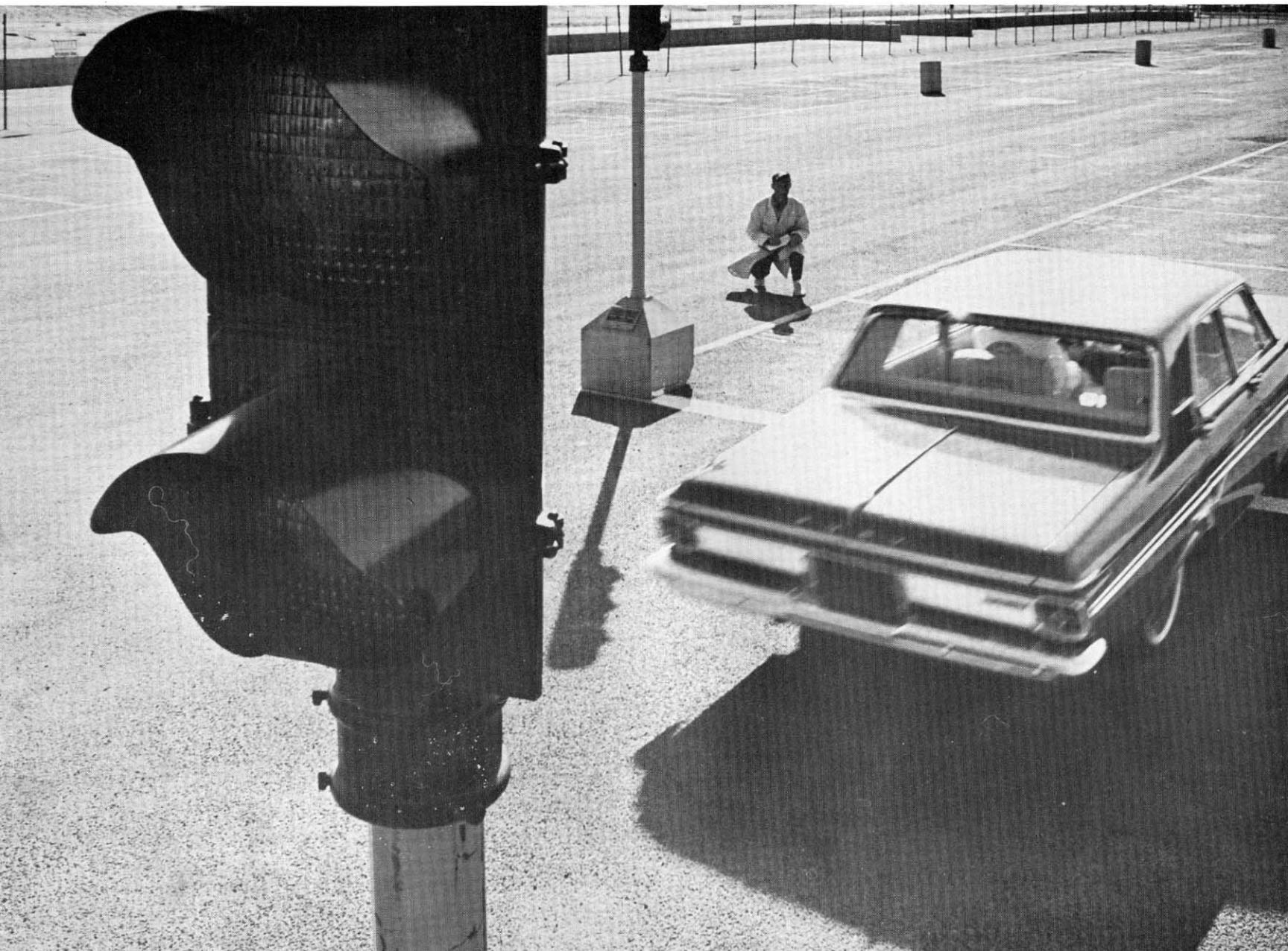
**EMERGENCY STOP** This is a test of braking ability. Each car races down the backstretch until it reaches a speed of 60 miles per hour. At that instant, the driver hits the brakes. NCTI officials arrive at the results by measuring the skid marks from one end to the other. After three runs for each car, with a different driver at the wheel for each run, the official average figures give Ford its
