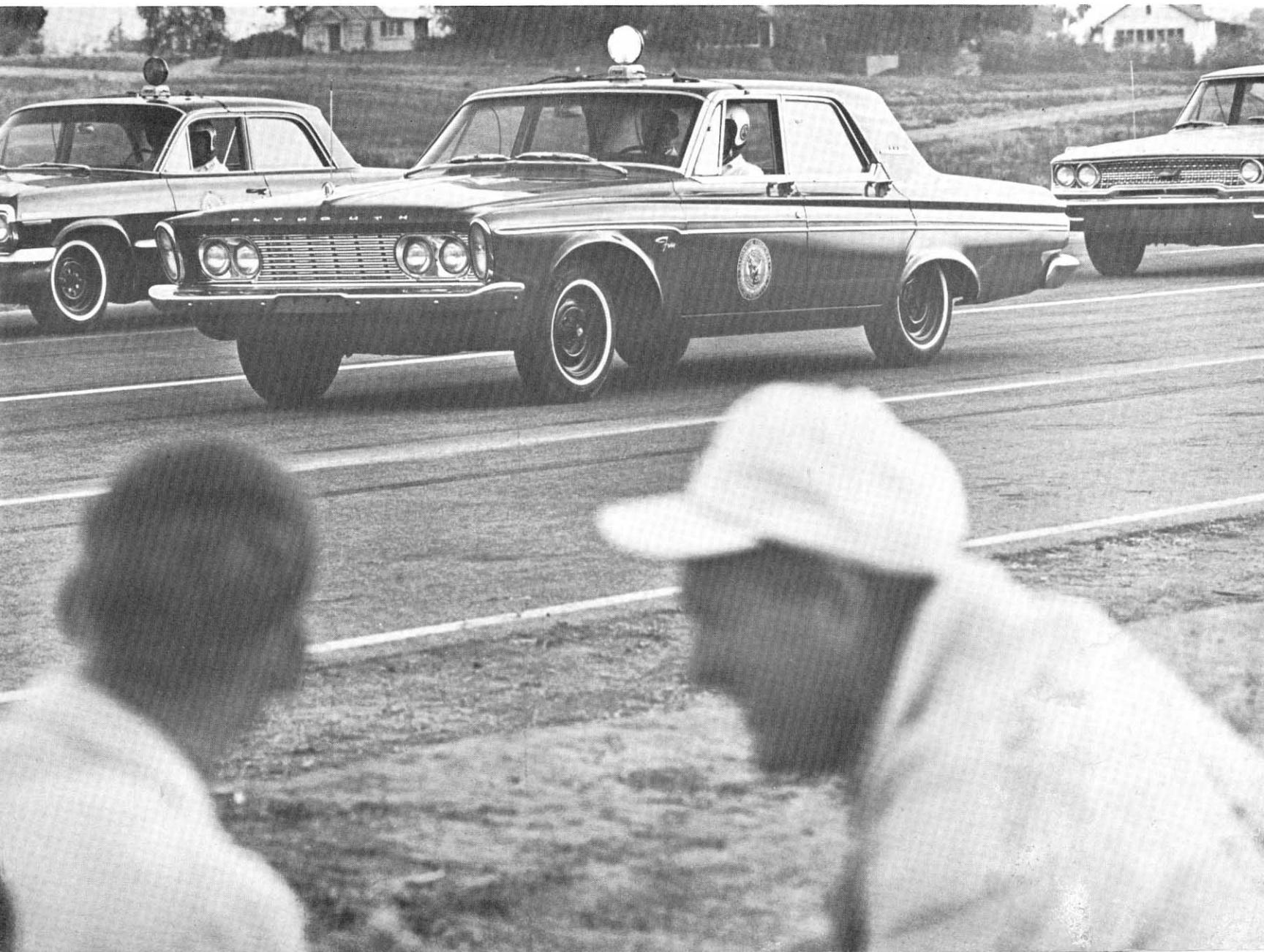
**QUARTER-MILE RUN** Here the tempo picks up. Another test of acceleration from a standing start, but this time over a longer stretch. A car needs more than quick response here; it needs stamina as well. Electronic equipment is ready on the backstretch. As each car crosses the finish line, the electric eye blinks and elapsed time is recorded automatically. Again, each car is run individually. Again, the three drivers get a crack at each car. Again, Plymouth comes home first,
