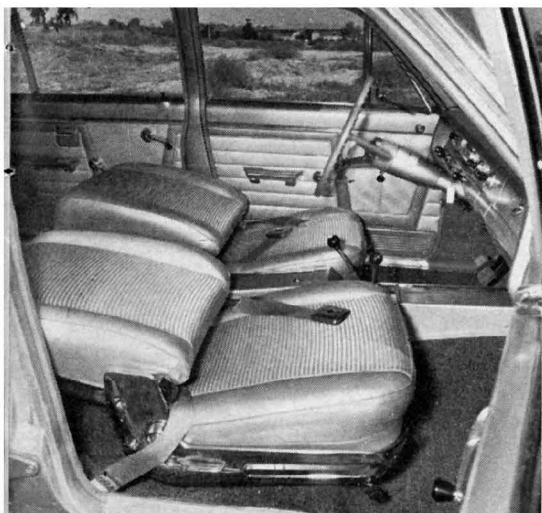
TILT-BACK seats are available with Twin Stick transmission option.
