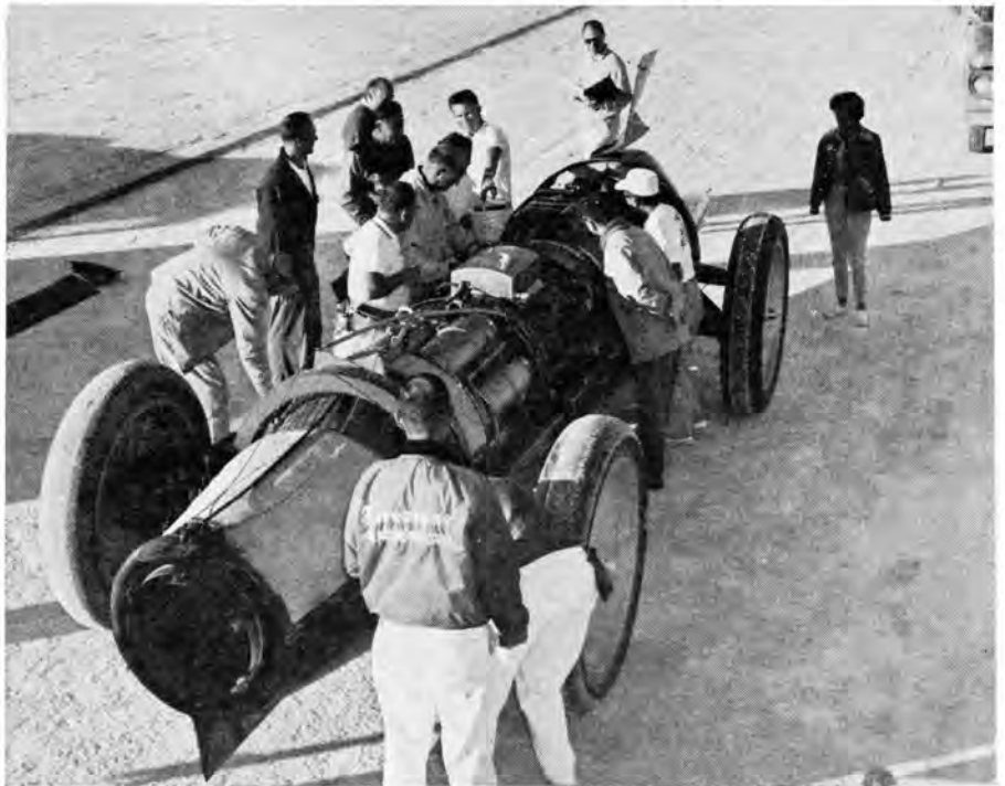
ABOVE —“Flying Caduceus” approaches track for LSR run. Note fin, added to improve directional stability at speed.
