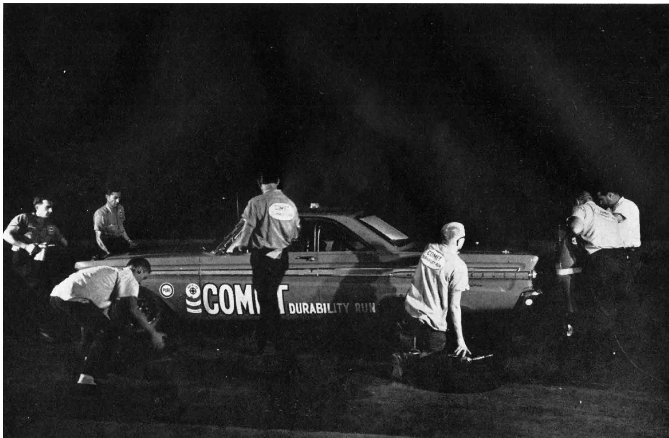
Every two hours, each car made a pit stop for additional fuel, water, and a change of drivers. Fast action by well trained and equipped pit crews kept stops down to 35-second average.
