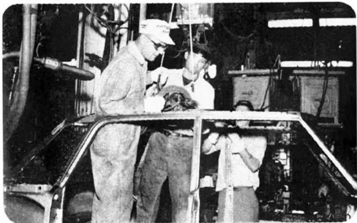
SPOT WELDER dangling from overhead is used at body form jig to tack roof cross brace into place, with some expert help.
