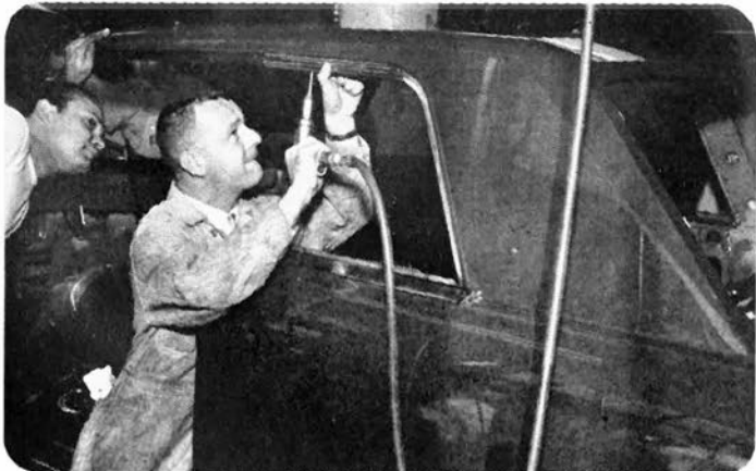
AFTER PAINT is sprayed and baked, first of the trim strips starts going into place. Deep concentration makes better job.
