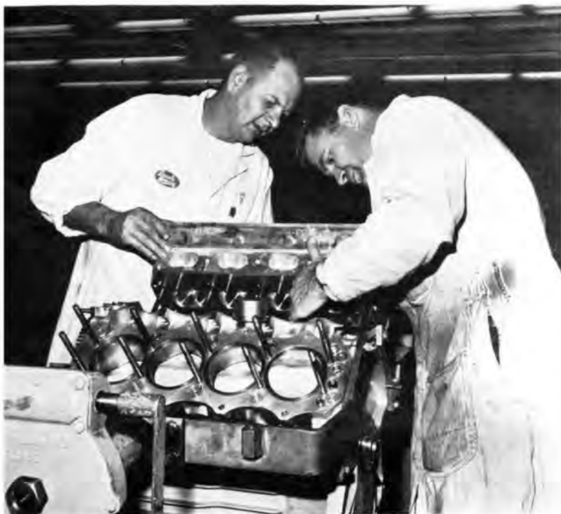
Back half of magnesium two-piece front cover closes off front of the crankcase, too. Water pump mounts below crankshaft, gear is on back side. Ball bearings in upper section of case are for shafts on each of the idler gears. LEFT - Bob Weeks, left, and Jerry Nine slide one of the heads over hold-down studs. Note that the exhaust ports, like the intakes, are large oval-shaped. Laminated steel O-rings seal cylinder gases; rubber O-rings, fluids.
