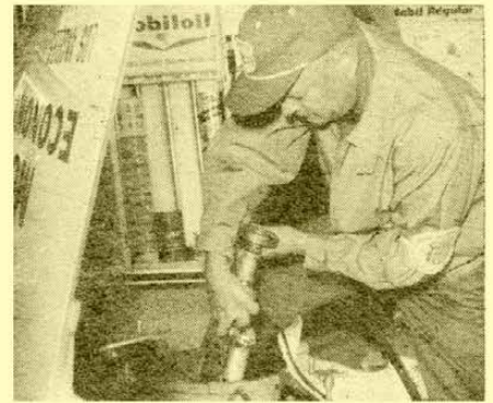
FUEL FOR run cars is measured into special tanks, then corrected to a specific temperature.
