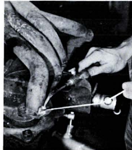
Here we see pipes being brazed to the flange plate. Headers are for 426 Dodge.
