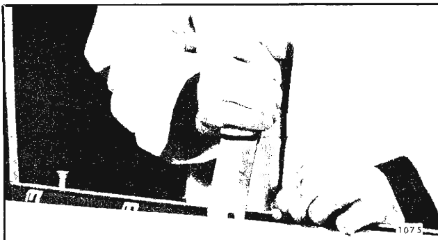
Fig. 5D15—Glass Run Channel Inner-Outer Strip Assembly Removal
