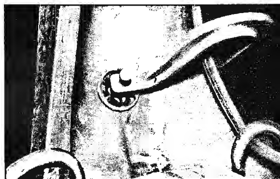
Fig. 13—Using Hot Patch Clamp
