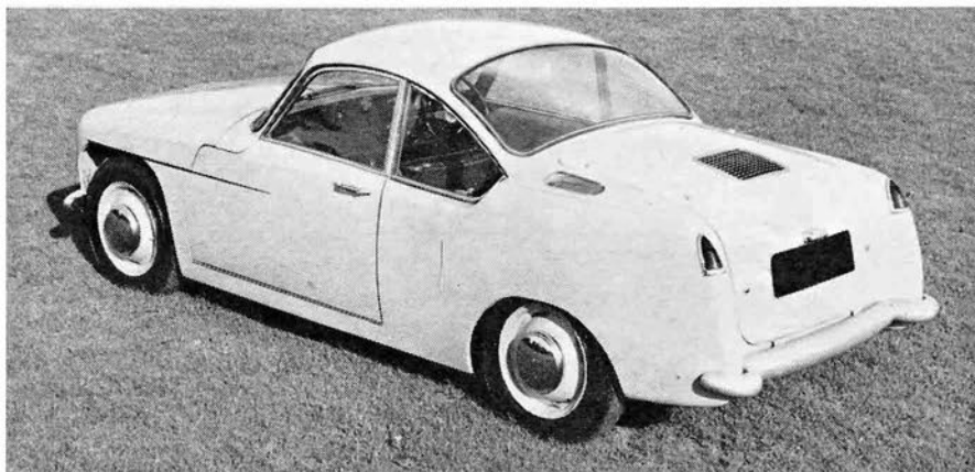
IN 1956, Rover's 4-wheel-drive turbine car appeared. Its rear axle was the prototype for the unit now on Rover 2000 cars.
