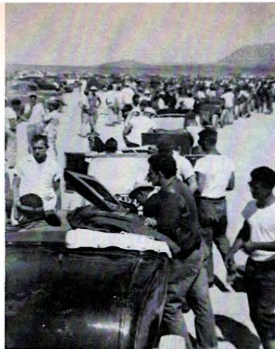
One of the first V-8 rods to really turn on was Karl Orr's modified, 134.40 mph. Modifieds ended at rear seat for body shell, tail piece or other fairings beyond this point classified car as a streamliner.
