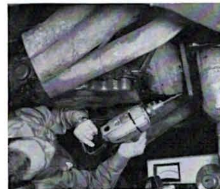
The electronic pickup will also detect vibrations at the rear of an engine in the car. Here an automatic transmission flywheel is being drilled to balance assembly.
