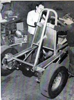
Above—Tom Smith (left) and Nash install the aluminum roll cage assembly. Unit attaches to channel frame through angle brackets at base of each leg with bolts. Team made almost entire chassis assembly of aluminum and stainless steel to keep weight down. Bronco tips scales at 1400 pounds.
