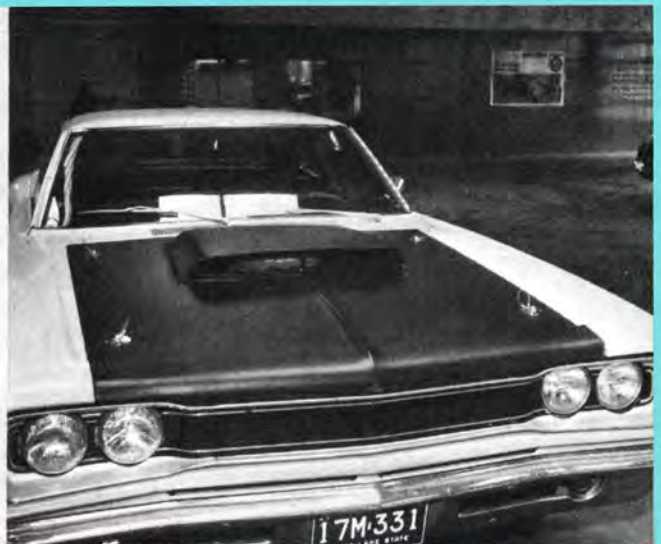
The new-old switcheroo from Chrysler Corporation this half-year is tri-power. Trio of Holley two-barrels go beneath 'glass hood.
