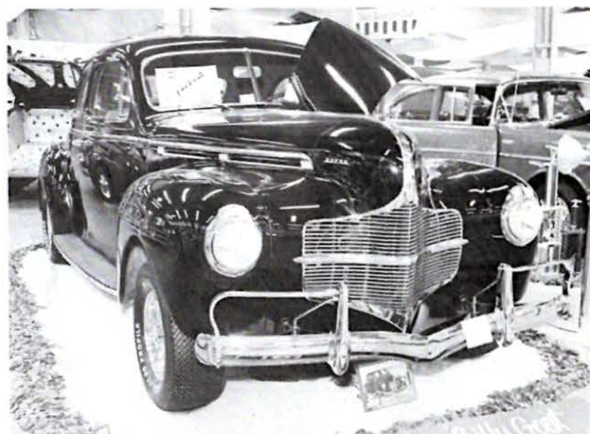
Sort of a rare item is this 1940 Dodge Business Coupe. Power is supplied by 307 Chevy mill with 310 heads. Tranny is Powerglide. Owner is Graham Alvey from Valley Station, Ky.
