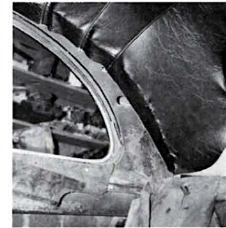
The liner is tacked and the wrinkles are worked out from the center toward the front or rear, as you go.
