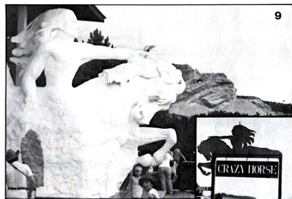
Since both Herby and myself had been to Mount Rushmore previously, we chose to stop at the construction site of Mr. Korczak's Crazy Horse Monument near Custer, South Dakota. Unbelievable! The mountain in the background will some day look like the sculpture.
