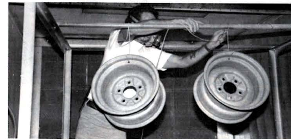
Dick electrically grounds the wheels before applying the powder.
